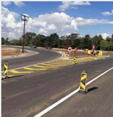
P156 road works about to be completed in Vanderbijlpark
